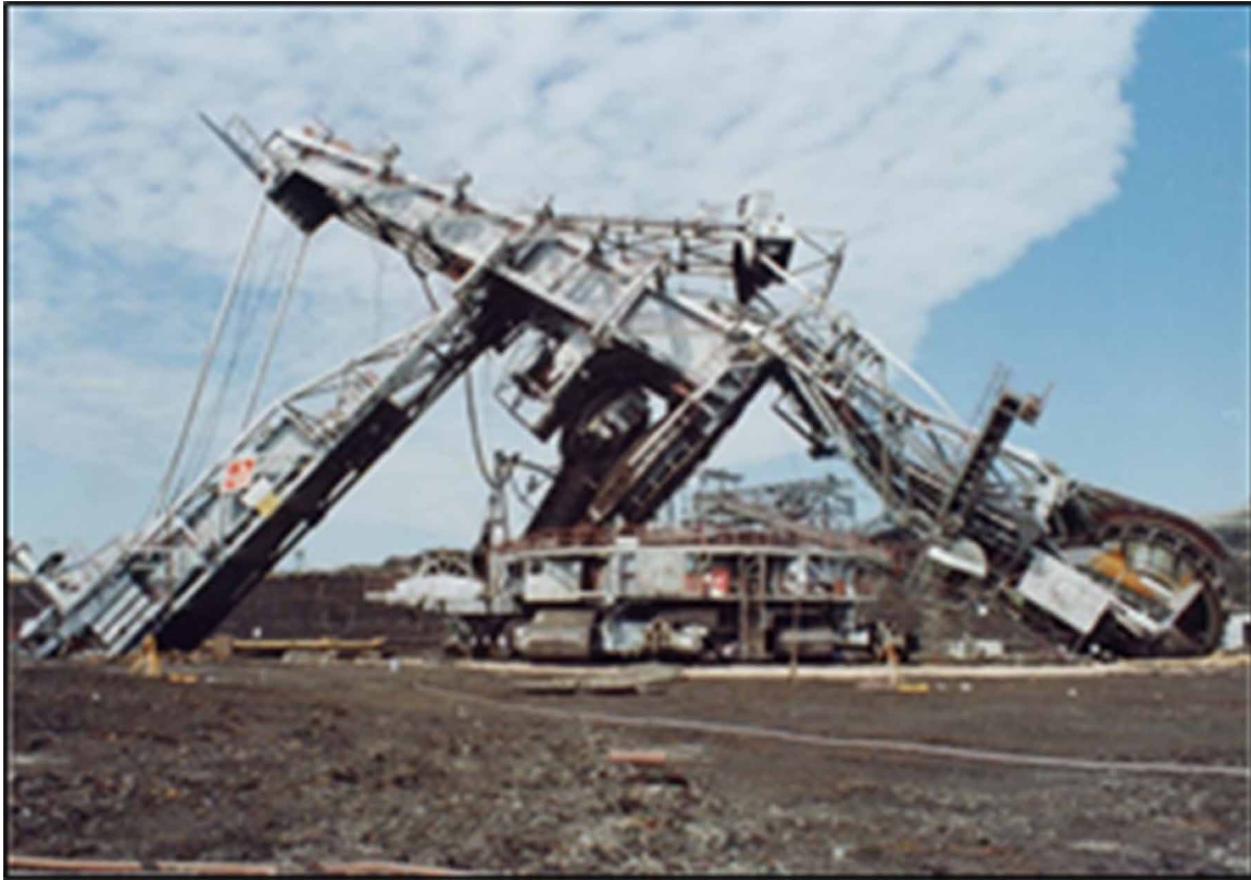
Figure 8. SchRs 630 after catastrophic failure
